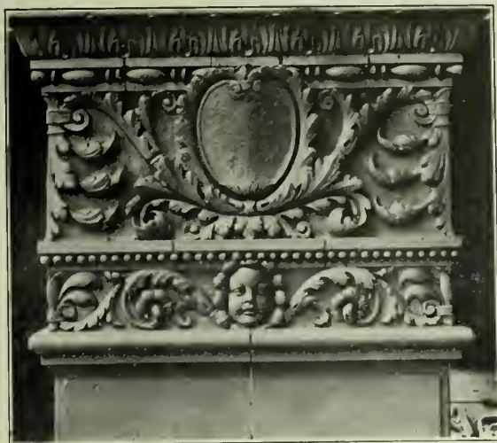
CAPITAL EXECUTED IN TERRA COTTA BY THE ATLANTIC TERRA COTTA COMPANY. McKim, Mead & White, Architects.
